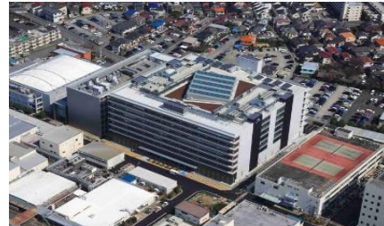
Solar panels installed on the roof of the R&D Labs (Japan)
