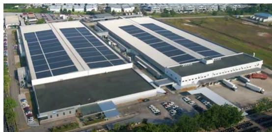
Konica Minolta Business Technologies (Malaysia) and roof-mounted solar panels
